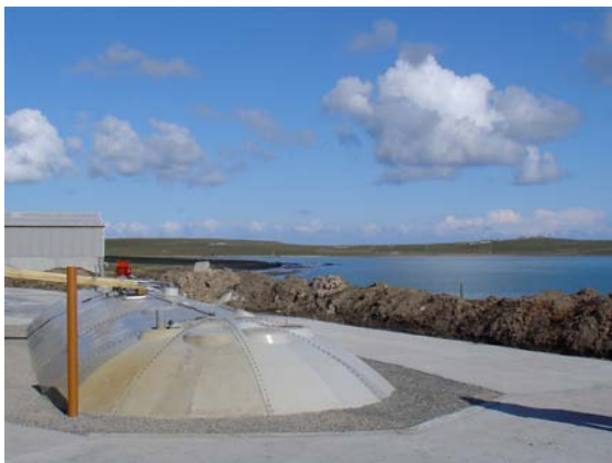
Westray anaerobic digester, Heat & Power Ltd.
