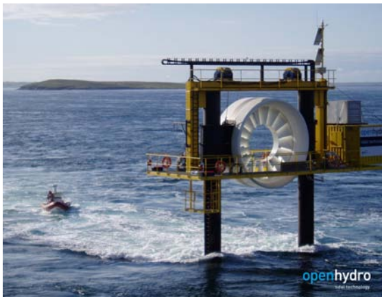
OpenHydro tidal turbine, installed at EMEC.
